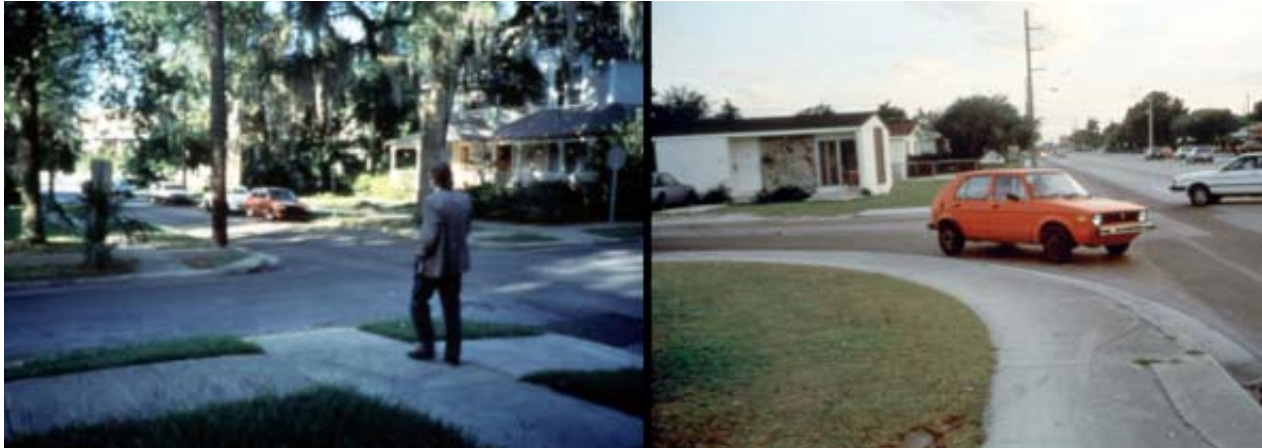
Compared to traditional tighter corners, large curb radii at intersections broaden crossing distances and encourage speeding.
