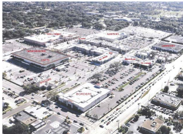
The Winter Park Mall was transformed into a main street configuration while retaining its anchor buildings.
