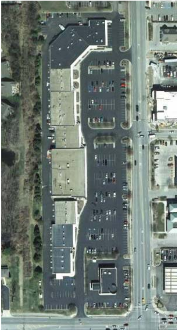
The current layout of the strip center, with buildings entirely set back behind parking.
