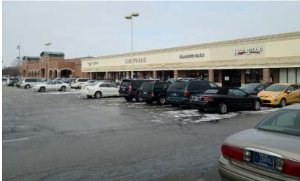
Merchants' Square is currently characterized by single-story retail buildings enfronted by large parking lots.
