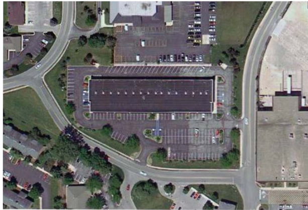
This strip center south of the Post Office has a history of high vacancy.
