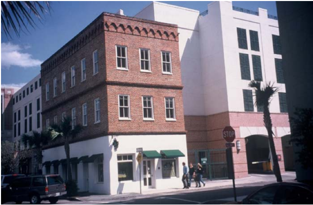
Only a narrow building is needed to hide a large parking garage from the sidewalk.
