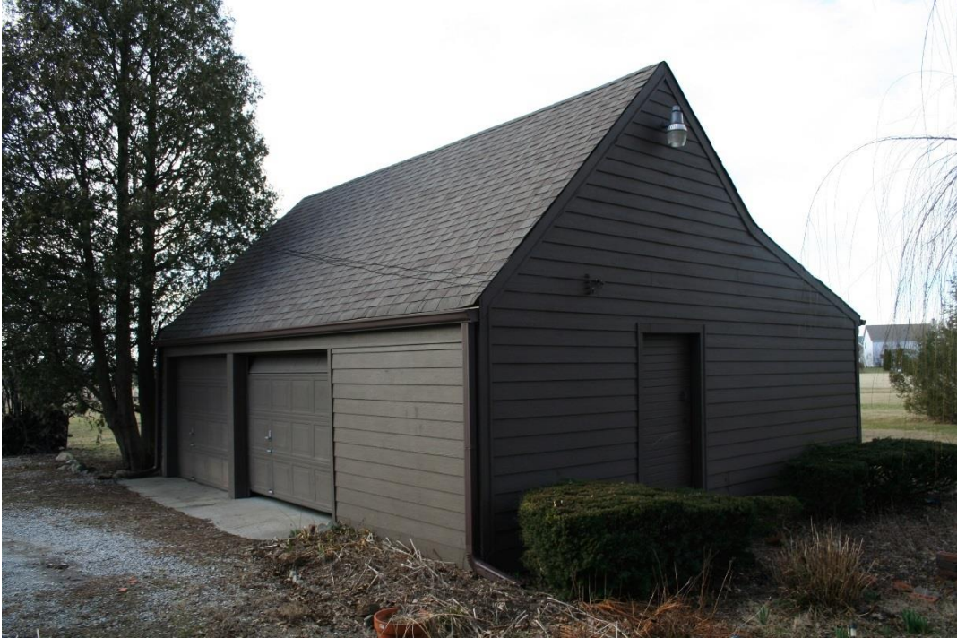
Appendix 1, Figure 6: Garage, south and east facades, looking northwest
