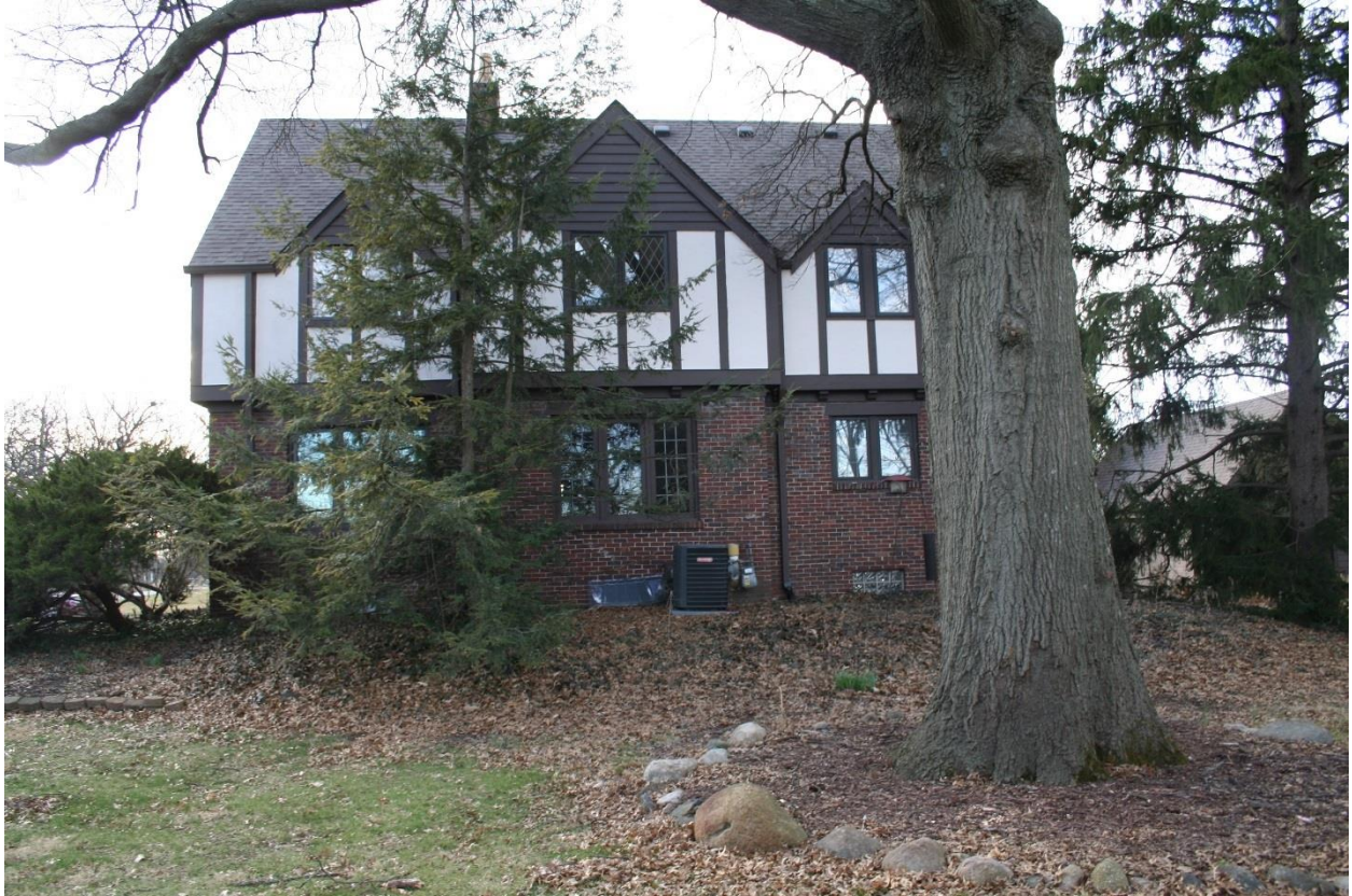
Appendix 1, Figure 4: East façade, looking west
