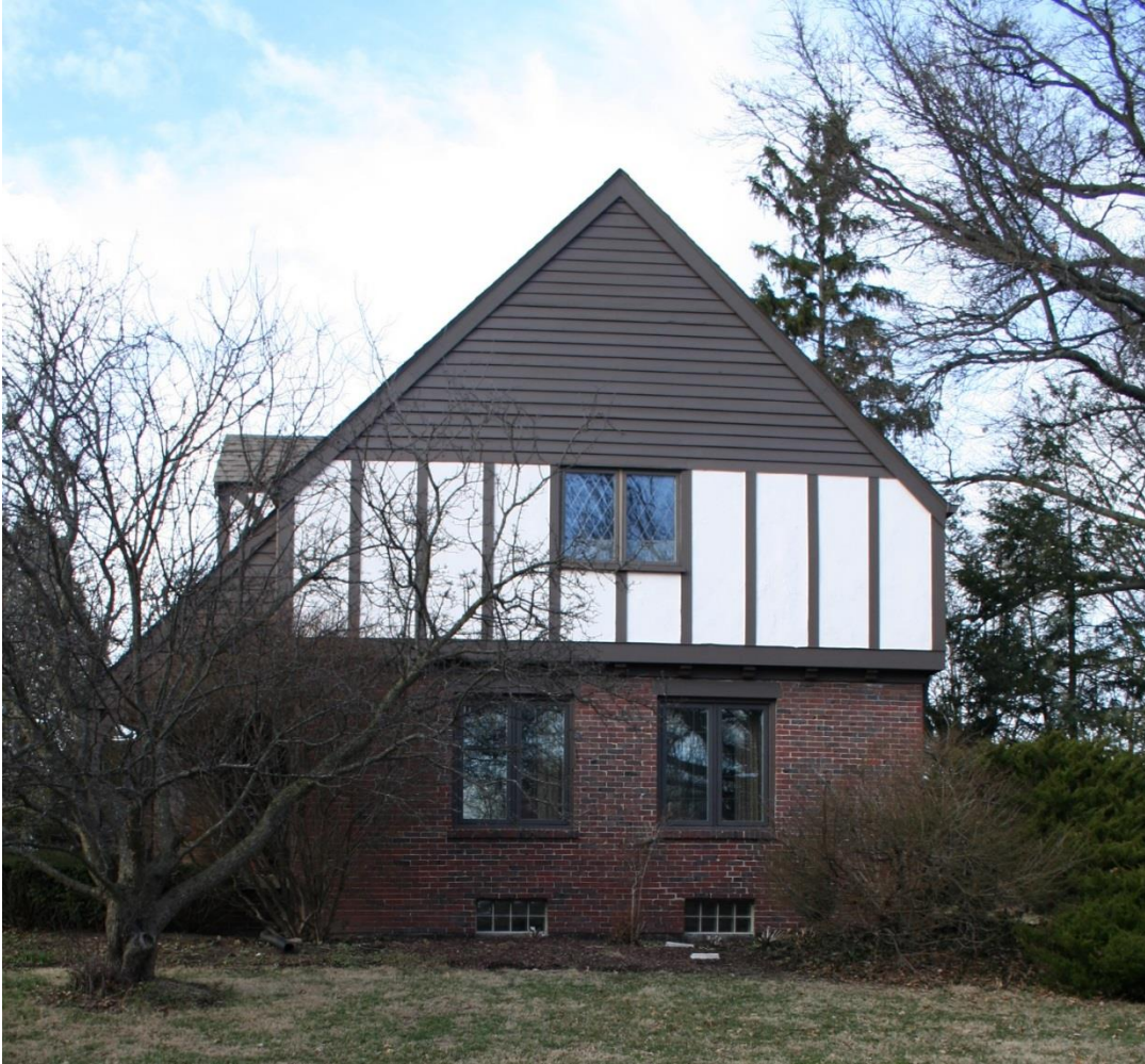
Appendix 1, Figure 3: South façade, looking north
