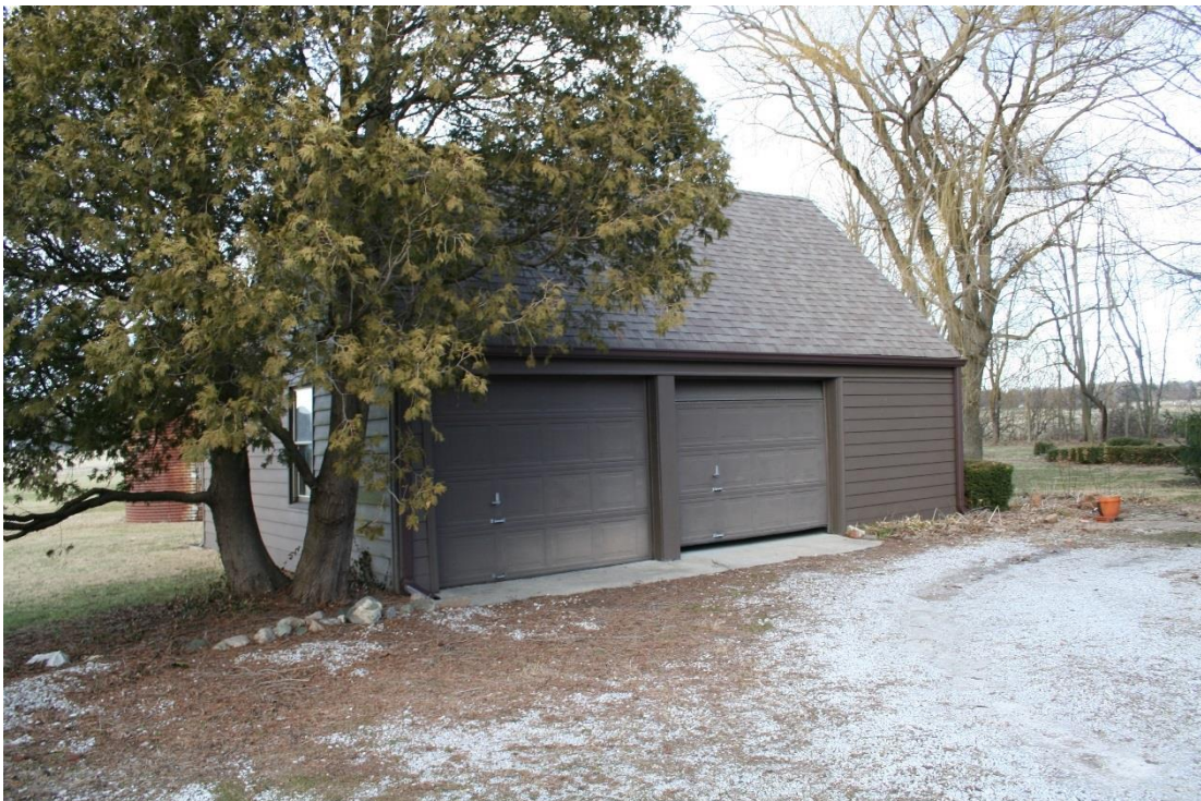
Appendix 1, Figure 7: West and south facades, looking northeast
