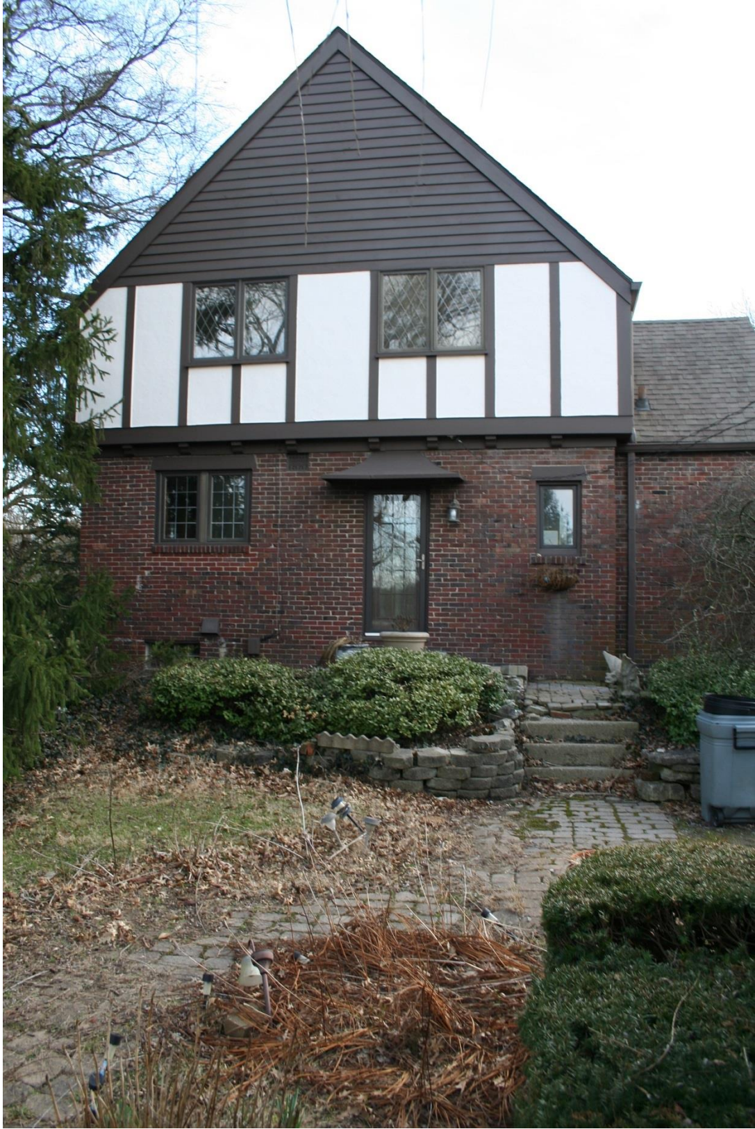
Appendix 1, Figure 5: North façade, looking south
