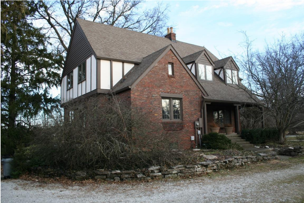
Appendix 1, Figure 1: West façade, looking southeast
