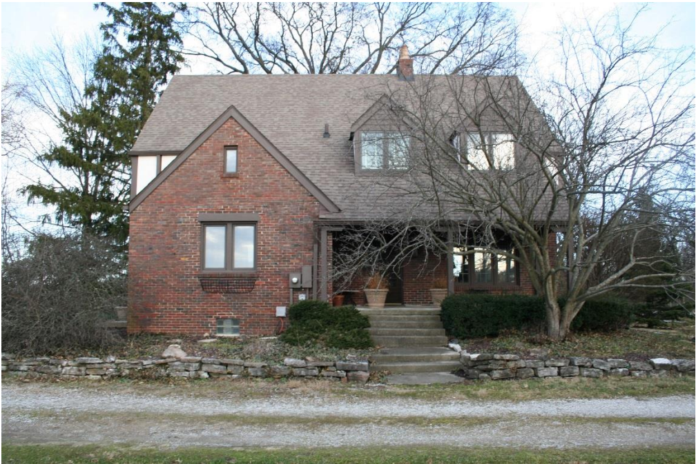
Appendix 1, Figure 2: West façade, looking east
