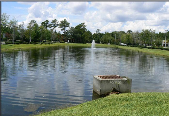
A detention pond and outlet control structure
