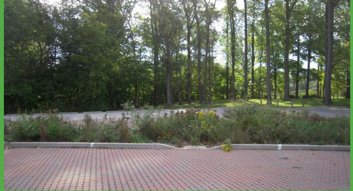
Porous paving units allow stormwater to infiltrate, thus replenishing groundwater and reducing the amount of pollution to the nearby stream.
