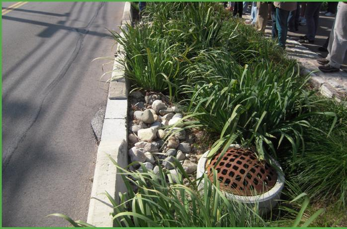
This roadside swale infiltrates water but also has an overflow drain to capture water during larger storms.
