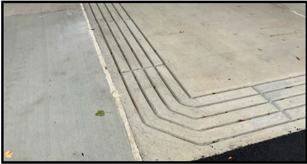
3 – Photo example of Positive Limiting Barrier (stormwater BMP and containment) at dispensing area.
