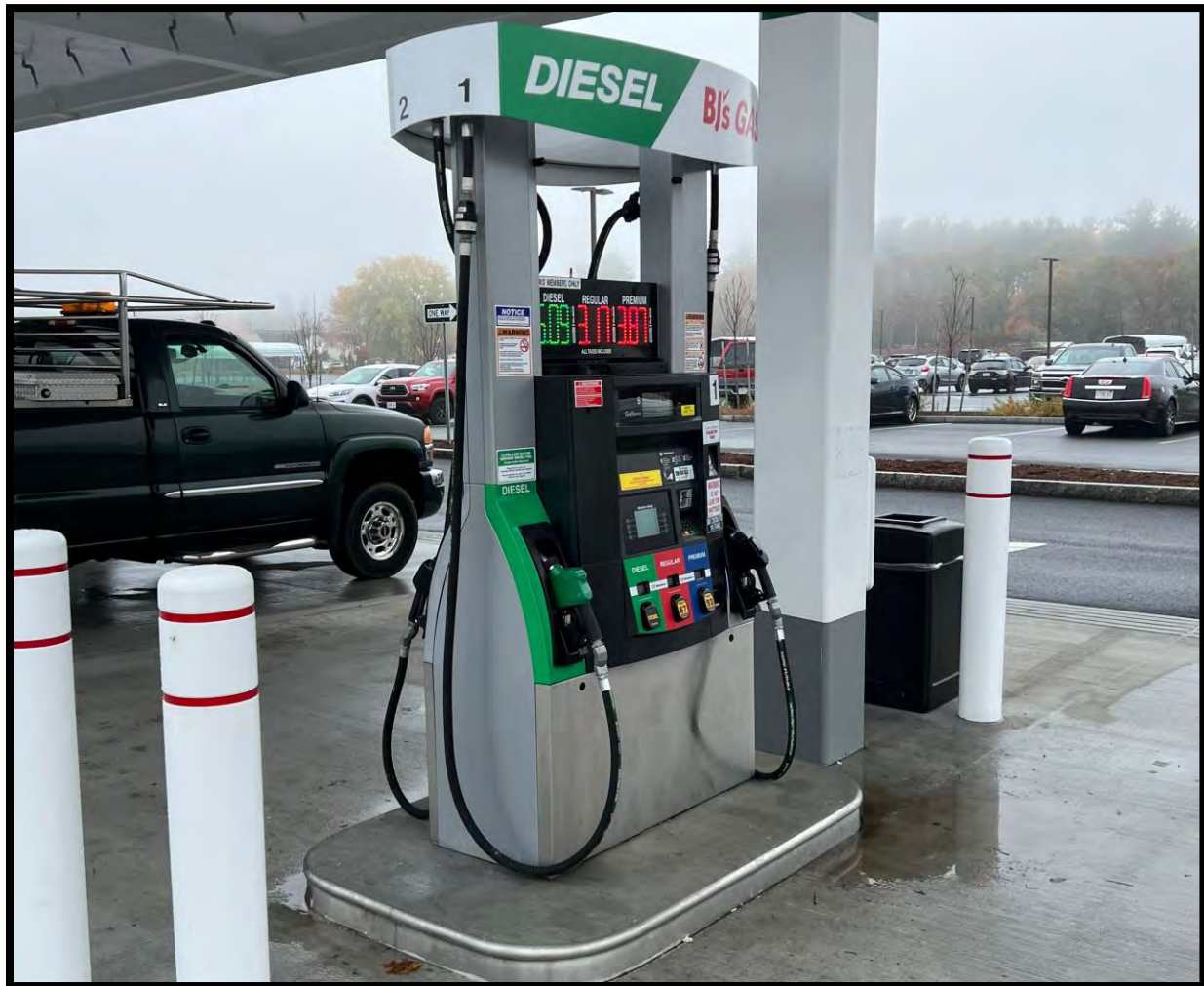
5 – Photo example of Continental Futura “Low Perm” hoses installed at a BJ's Gas Station to provide added air quality protection.
