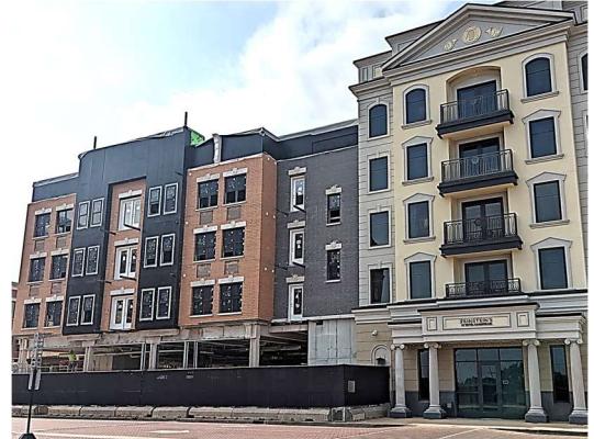
Currently under construction
