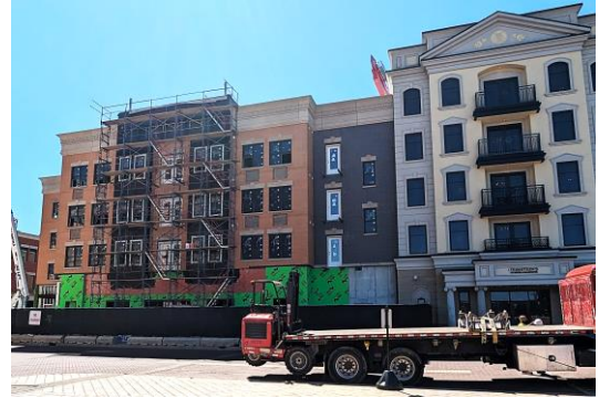
Currently under construction
