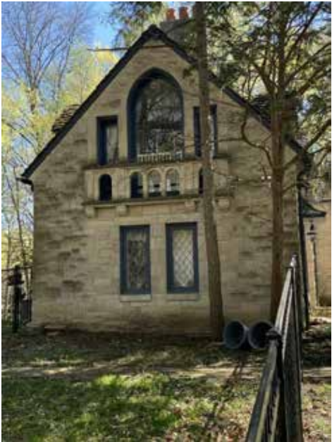
Appendix 1, Figure 2: North façade
