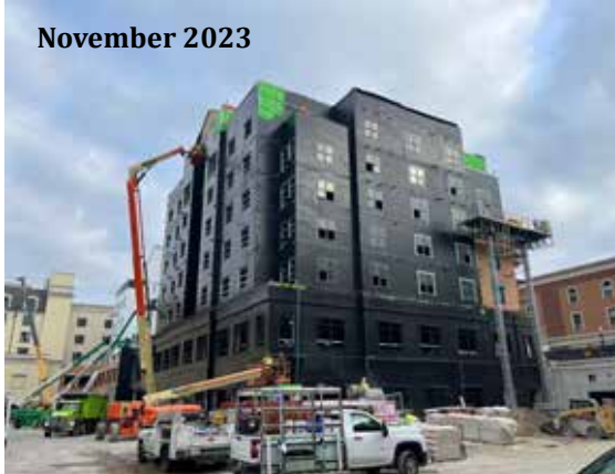
Currently under construction
