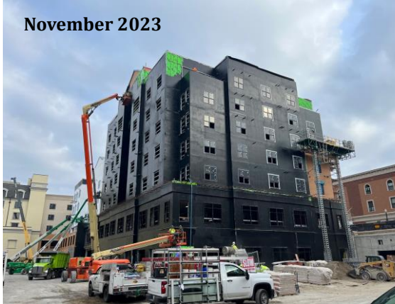
Currently under construction
