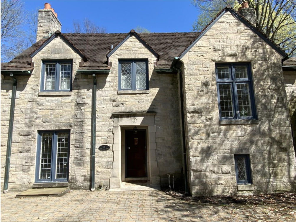
Appendix 1, Figure 1: West façade
