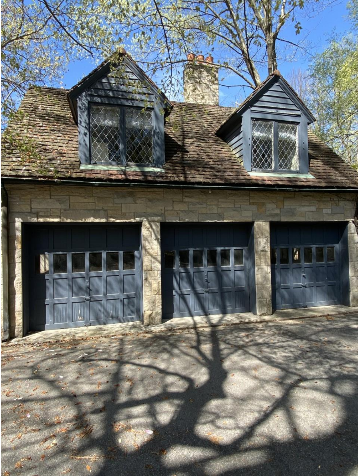
Appendix 1, Figure 3: South façade
