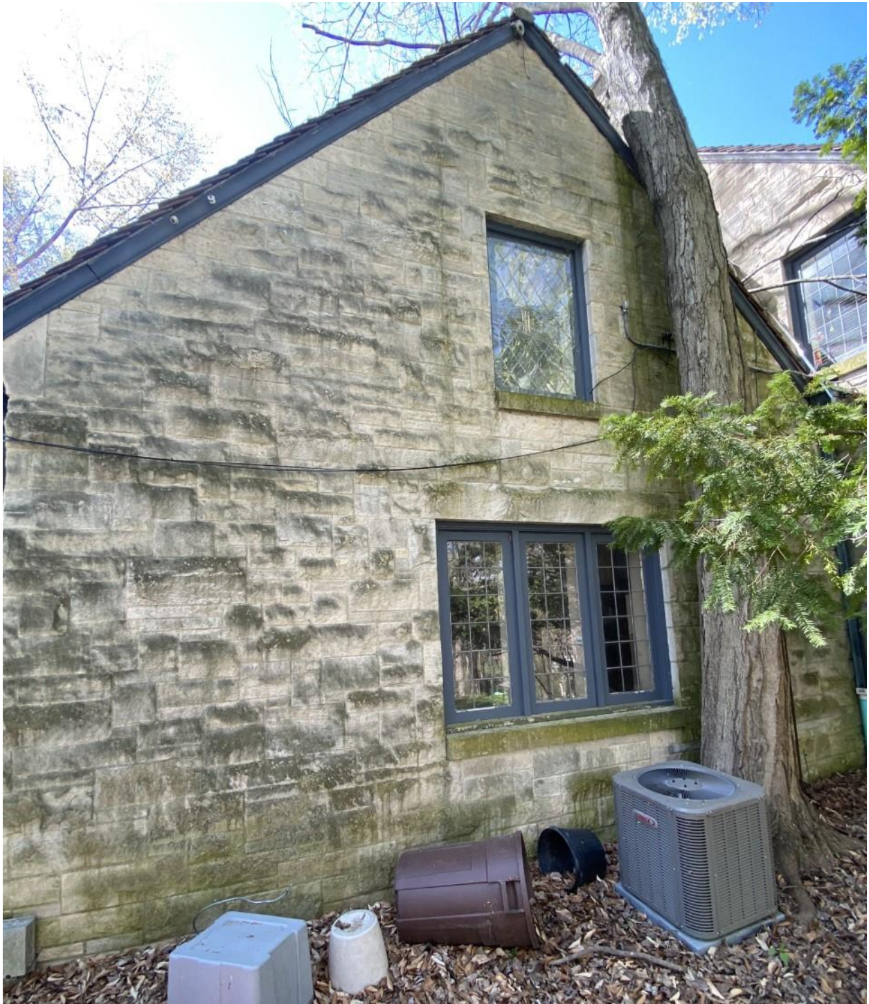
Appendix 1, Figure 4: East façade
