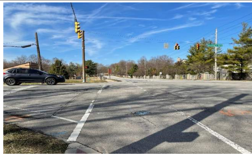
Photo 25. Looking west toward 106 th Street from the southeast corner of the intersection.
