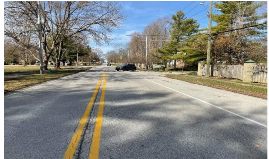
Photo 48. Looking west down 106 th Street, approximately 0.16 mile west of the intersection.
