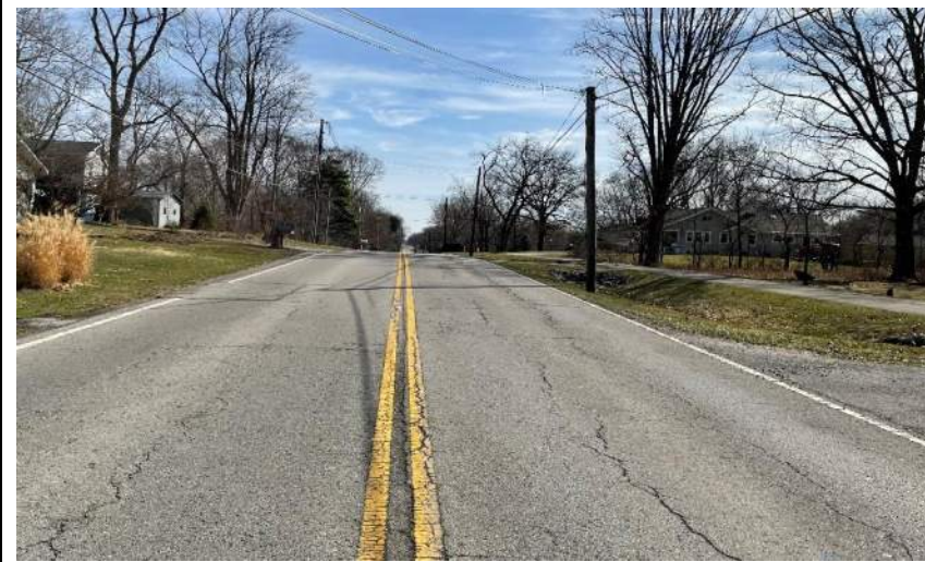
Photo 19. Looking east up E. 106 th Street, approximately 0.10 mile east of the intersection.
