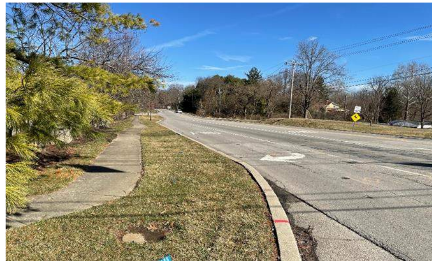
Photo 35. Looking north down Westfield Blvd. from the northwest corner of the intersection.
