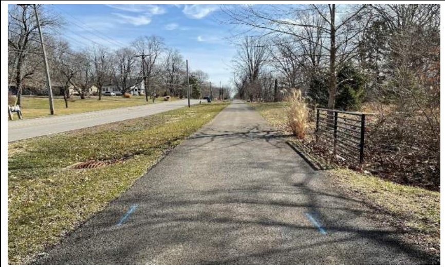
Photo 22. Looking east along the south side of 106 th Street, approximately 0.05 mile east of the intersection.
