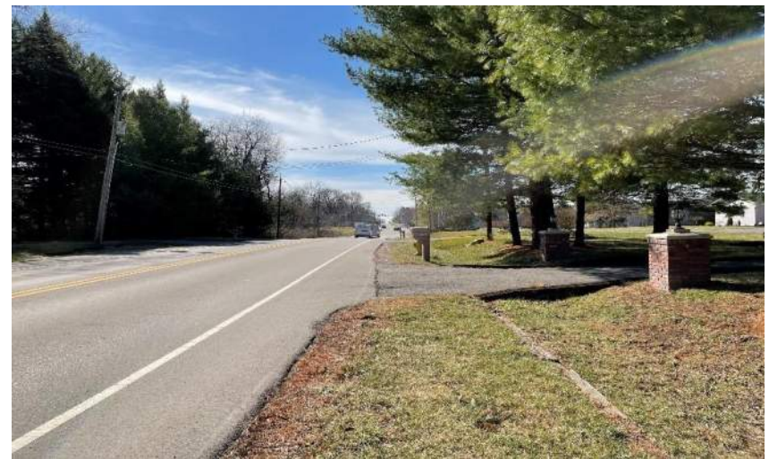
Photo 4. Looking south along the west side of Westfield Blvd., approximately 0.14 mile north of the intersection.
