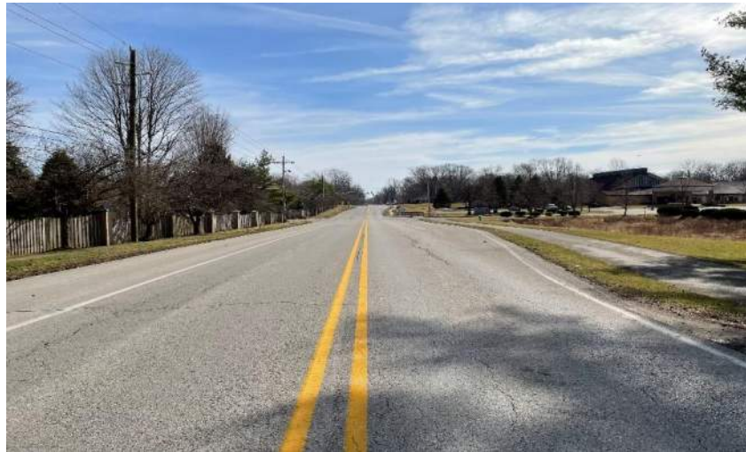
Photo 47. Looking east up 106 th Street, approximately 0.16 mile west of the intersection.
