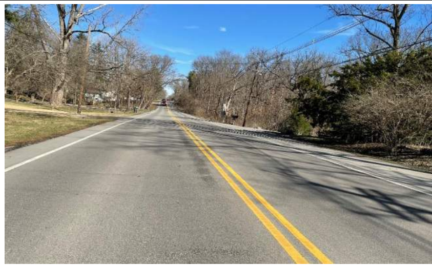
Photo 1. Looking north up Westfield Blvd., approximately 0.16 mile north of the E. 106 th Street and Westfield Blvd. intersection.
