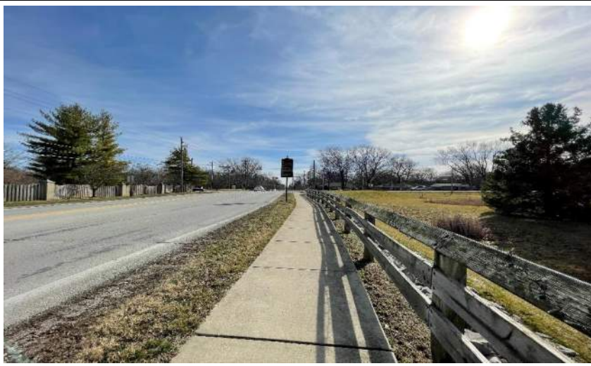
Photo 37. Looking east along the south side of 106 th Street, approximately 0.06 mile west of the intersection.
