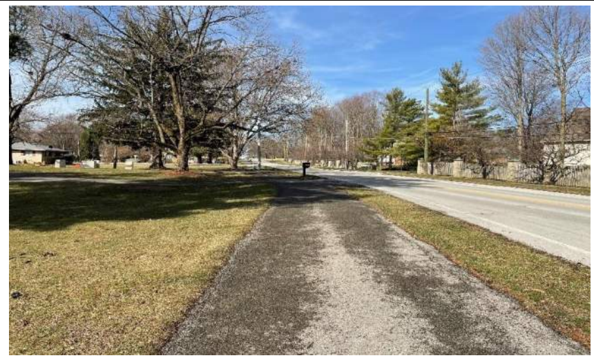
Photo 46. Looking west along the south side of 106 th Street, approximately 0.12 mile west of the intersection.
