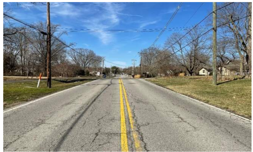
Photo 20. Looking west down 106 th Street, approximately 0.14 mile east of the intersection.
