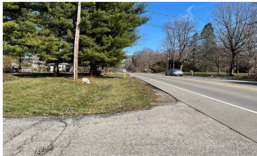
Photo 3. Looking north along the west side of Westfield Blvd., approximately 0.14 mile north of the intersection.
