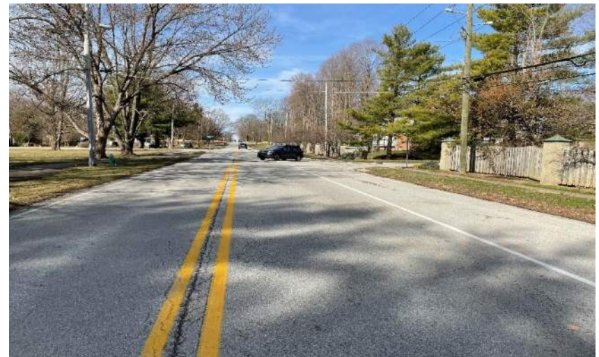
Photo 48. Looking west down E. 106 th Street, approximately 0.16 mile west of the intersection.
