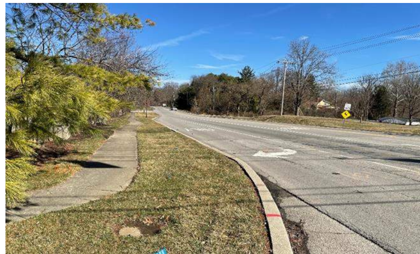
Photo 35. Looking north down Westfield Blvd. from the northwest corner of the intersection.
