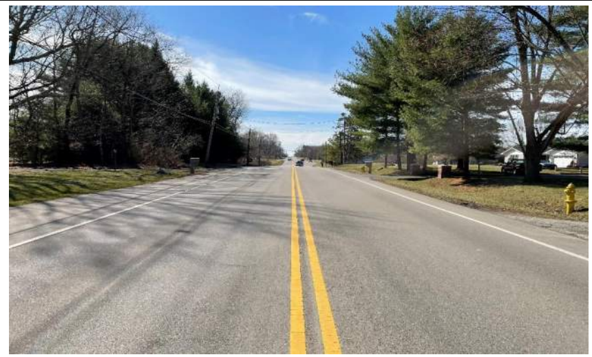
Photo 2. Looking south down Westfield Blvd., approximately 0.16 mile north of the intersection.
