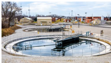
Figure 60. 2021 Wastewater Treatment Plant Expansion/One new final clarifier. Source: City of Carmel Utilities.
