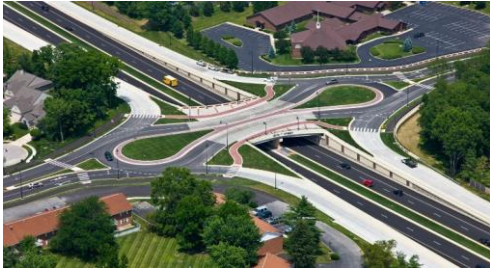
Figure 75. 126th street roundabout in Carmel, IN. Source: DOCS, 2023
