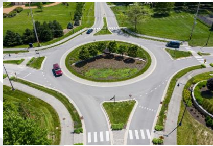
Figure 64. Roundabout in Carmel, Indiana. Source: Carmel Government official website.
