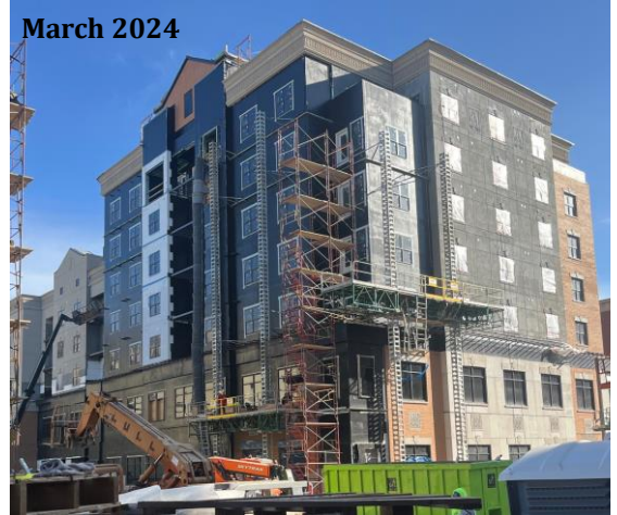
Currently under construction
