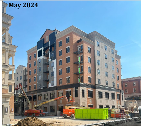
Currently under construction
