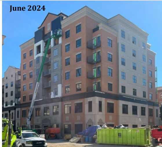
Currently under construction
