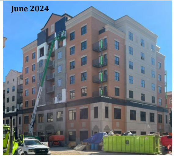
Currently under construction
