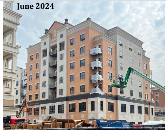
Currently under construction
