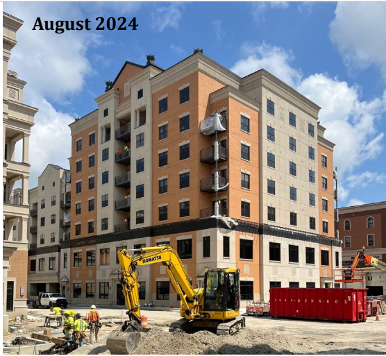
Currently under construction
