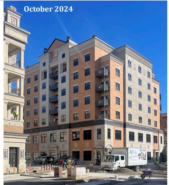
Currently under construction
