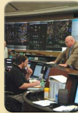
Midwest ISO control room
